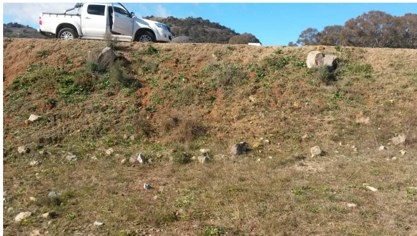
Photos 5 to 6 (above) – 18/7/14 – View of road fill and fill stockpiles on north-western side of the site.
